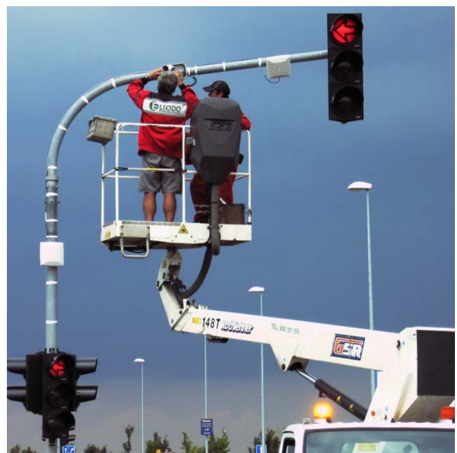
Installation of testing equipment on traffic lights
