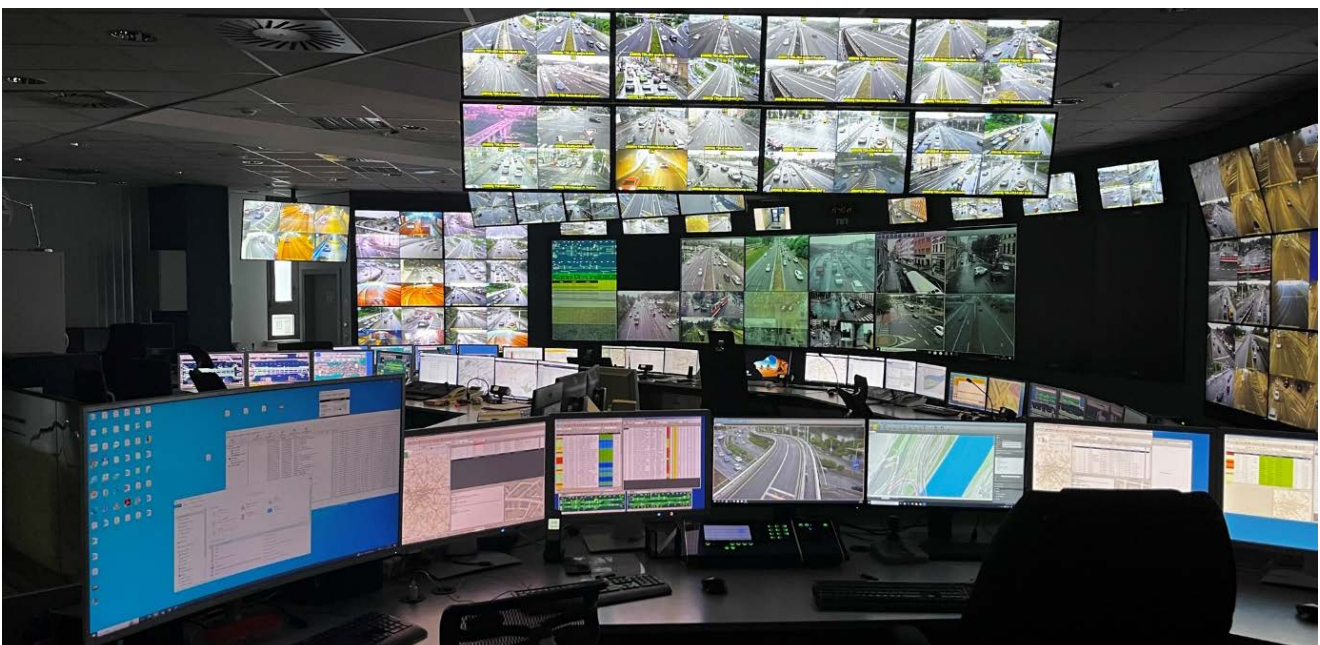
Main Traffic Control Center and the Traffic Information Center
